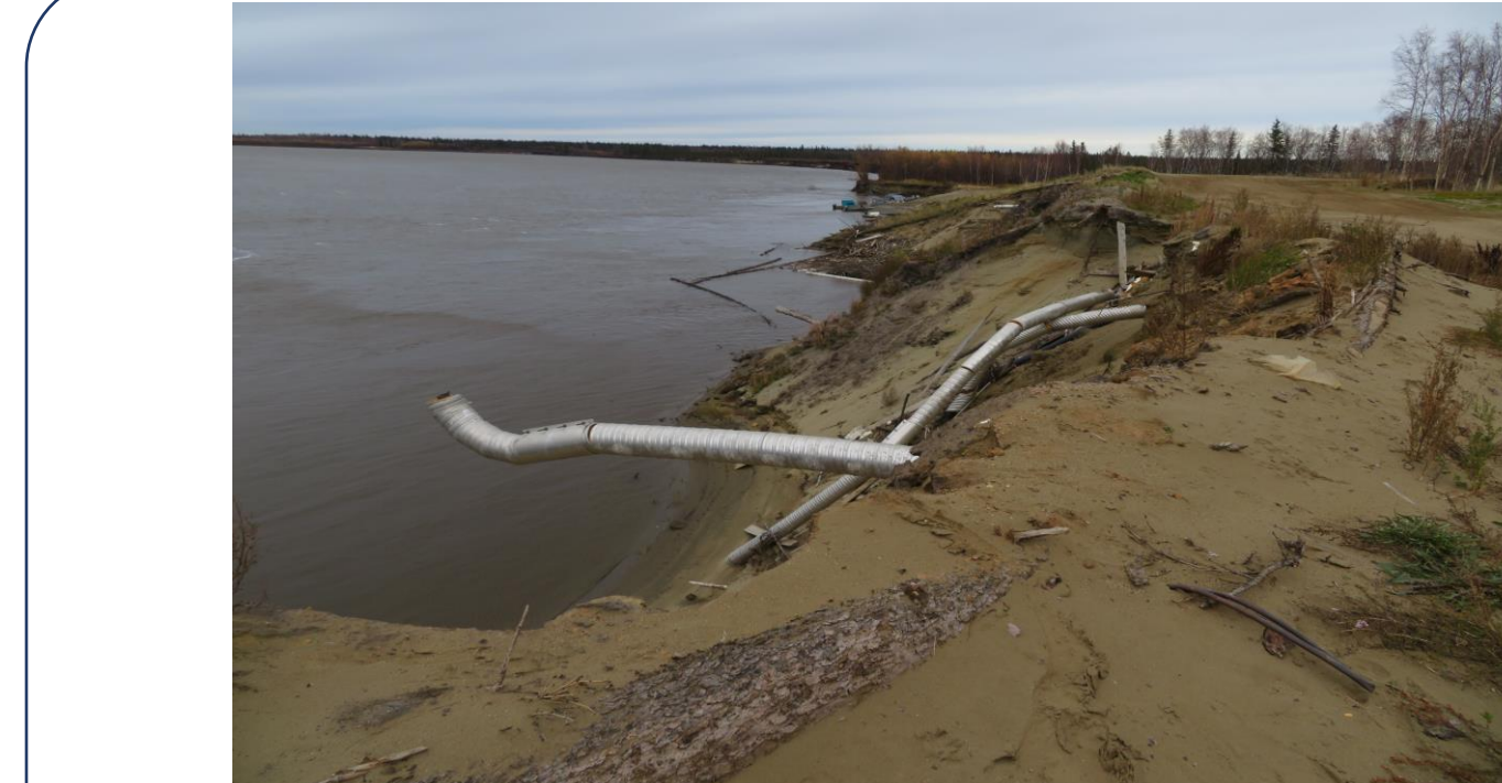
Fig 8: Huslia riverbank erosion and impacts to infrastructure. Sept 2022. Photo: Marie Lowe
